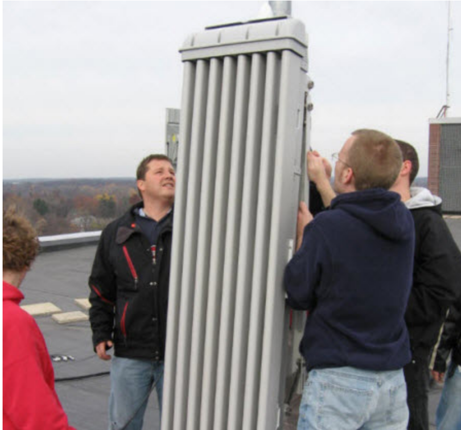
Ball State University Students Installing Outdoor WiMAX Antenna
