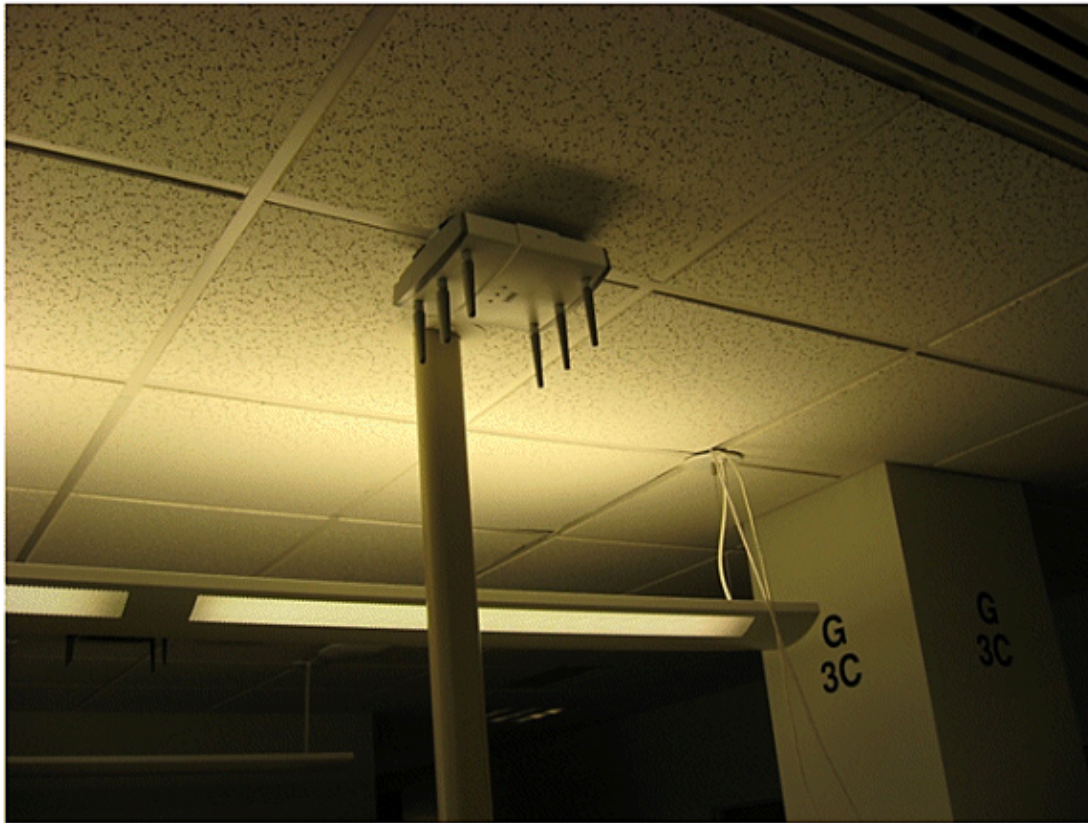
Figure 12: Poor AP Placement – AP Placed Near Physical Obstruction
