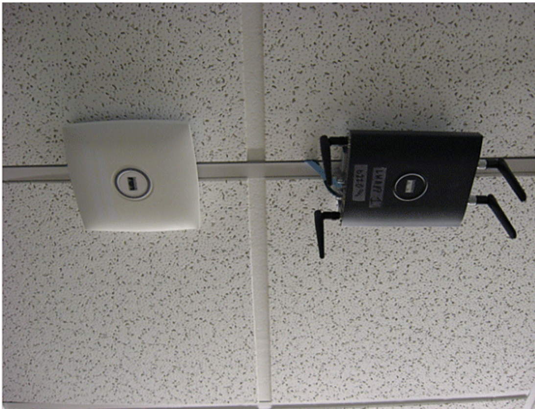
Figure 13: Poor AP Placement APs Placed Close to Each Other
