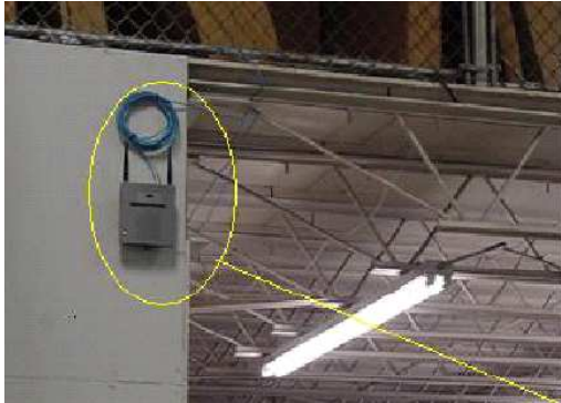
Figure D-3 AP and Antennas Mounted on a Wall, Away from I-Beams
