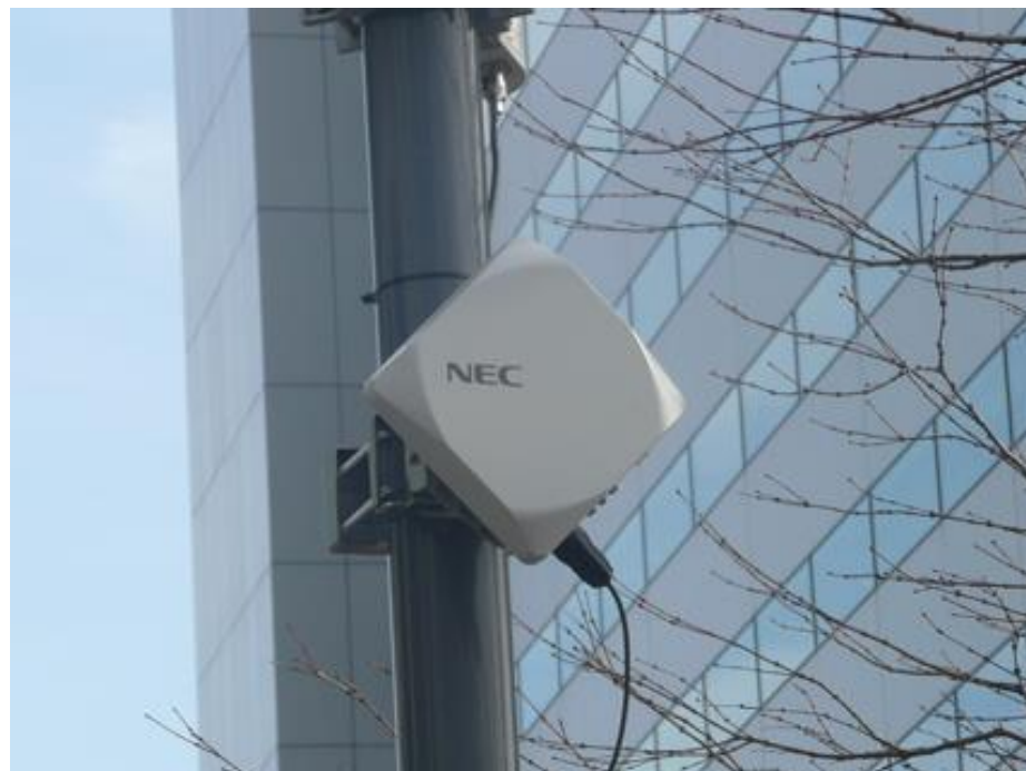
Figure 19. iPASOLINK SX 60 GHz microwave backhaul system for small cells. Source: NEC
