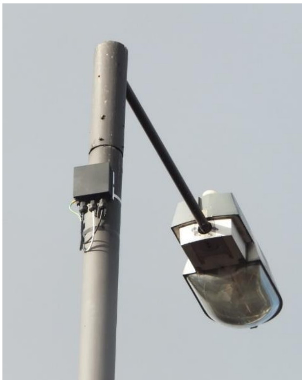
Figure 10. Siklu EtherHaul PTP radio mounted on a street lamp. Source: Siklu
